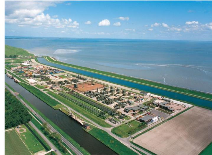
Three trunk lines, transporting hydrocarbon gas liquid mixtures from offshore gas and oil platforms, are landed at the Den Helder gas plant.
